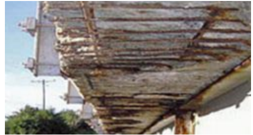
A bridge in Missouri that's in need of repair. (Missouri Department of Transportation)
